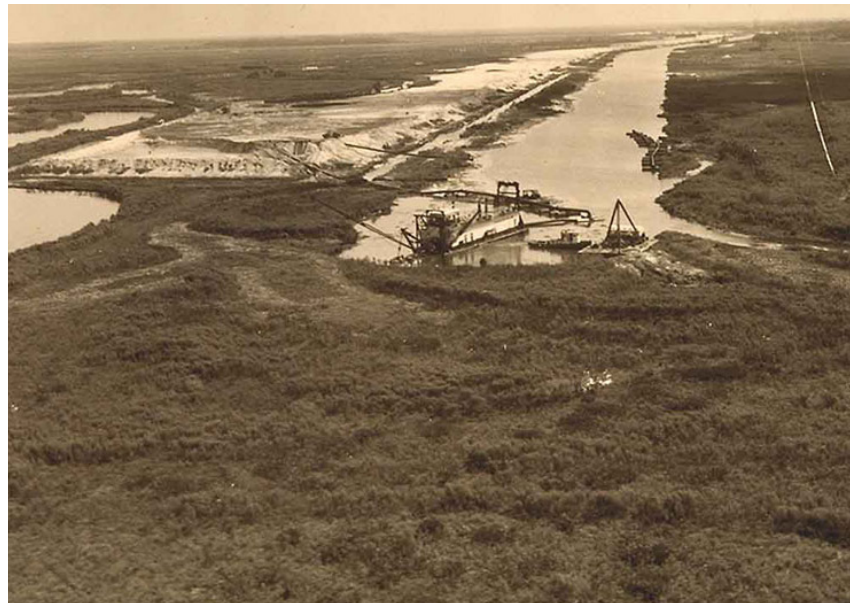
Channelization of the Kissimmee River PHOTO COURTESY OF FLORIDA ATLANTIC UNIVERSITY CORPS OF ENGINEERS
