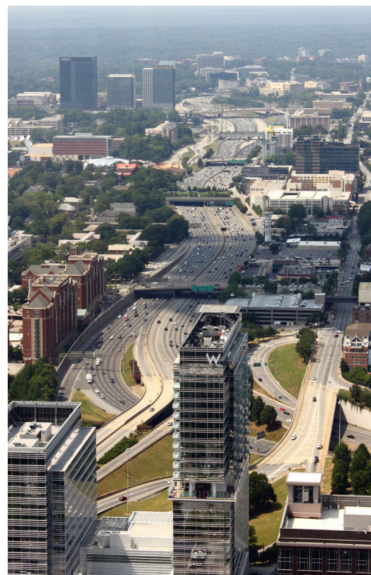
Dense development prevents expansion of the I-75/I-85 Connector in downtown Atlanta. Public transportation and surface street improvements can help alleviate congestion and provide local drivers with alternatives. (Flickr/muora)
