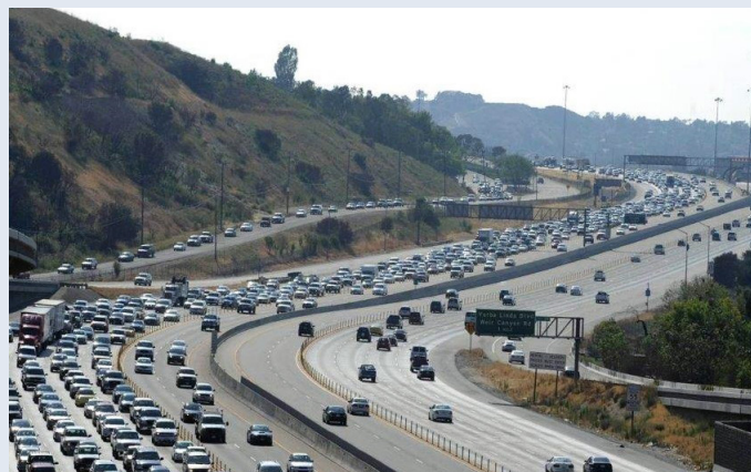
Express lanes allow traffic to move freely even as general travel lanes grind to a halt. (Orange County Transportation Authority)
